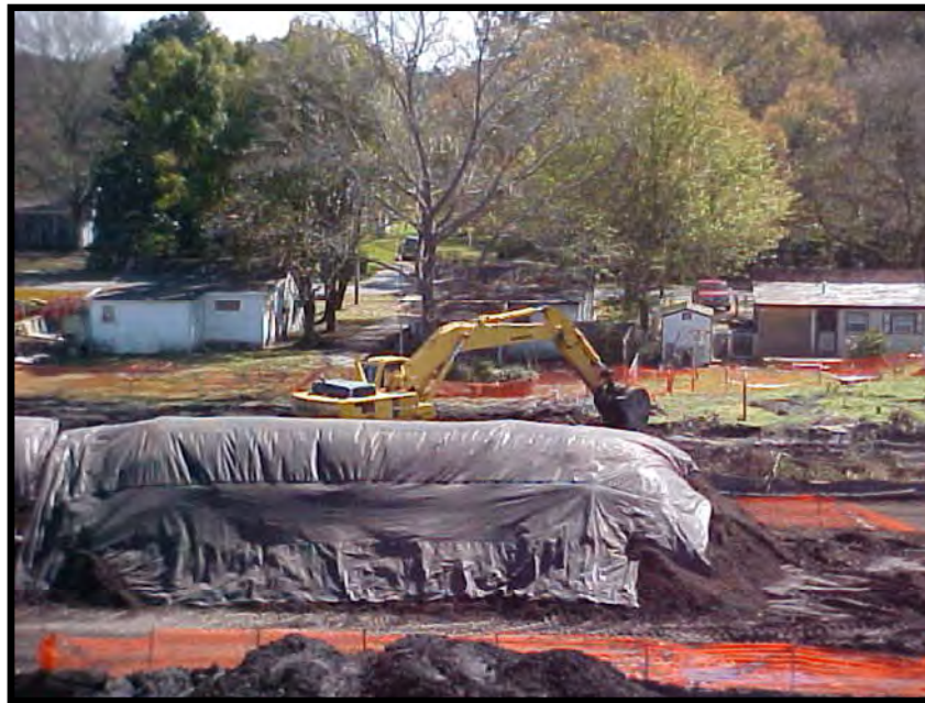
Figure 6. Stockpile Covered with Plastic Sheetting.
