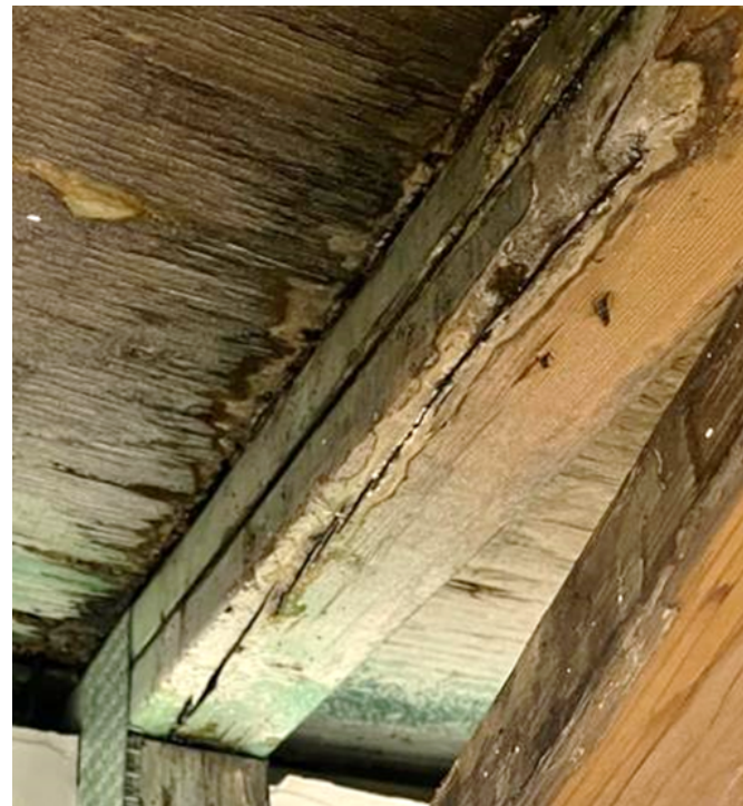
1 MEMBER SECTION LOSS S2 NTS
