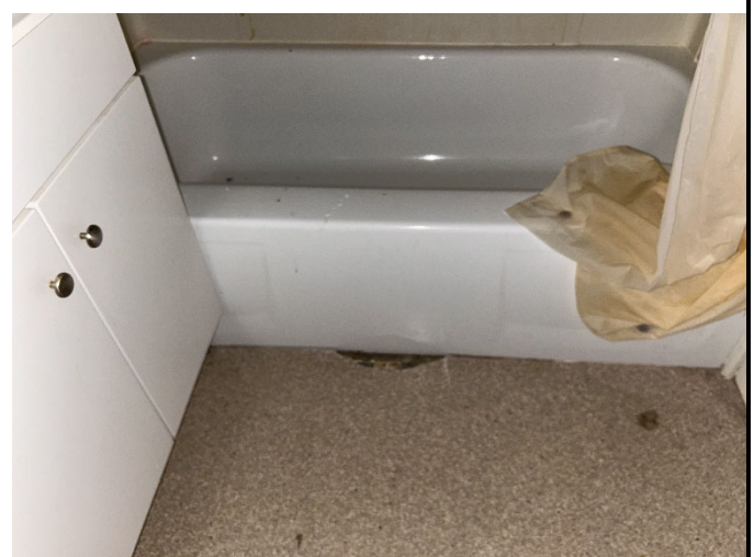
Photo 6. PACBM and PCBs sampling location, floor tile in bathroom – AS07/PCB07
