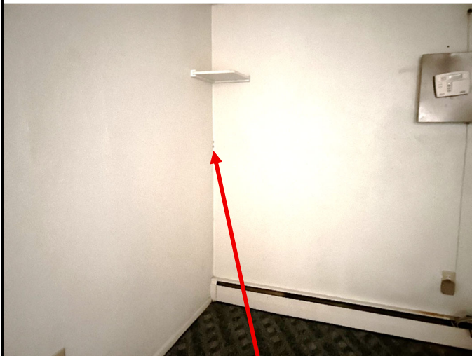
Photo 3. PACBM and PCBs sampling location, wall materials in Room 1 – Sample AS03/PCB03
