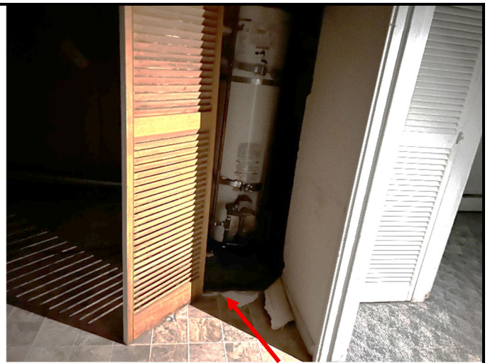
Photo 8. PACBM and PCBs sampling location, flooring materials in Kitchen – Sample AS111/PCB11
