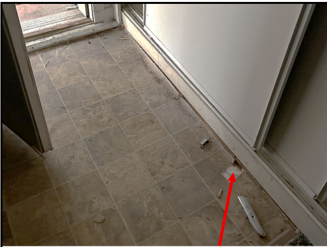
Photo 1. PACBM and PCBs sampling location, flooring material in entryway – Sample AS-01/PCB01
