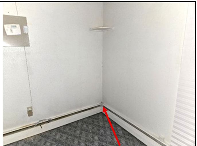
Photo 2. PACBM and PCBs sampling location, wall materials in Room 1 – Sample AS02/PCB02
